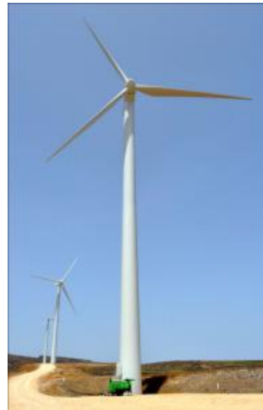
8 MW Wind Farm, in Sal, Cape Verde Under construction
