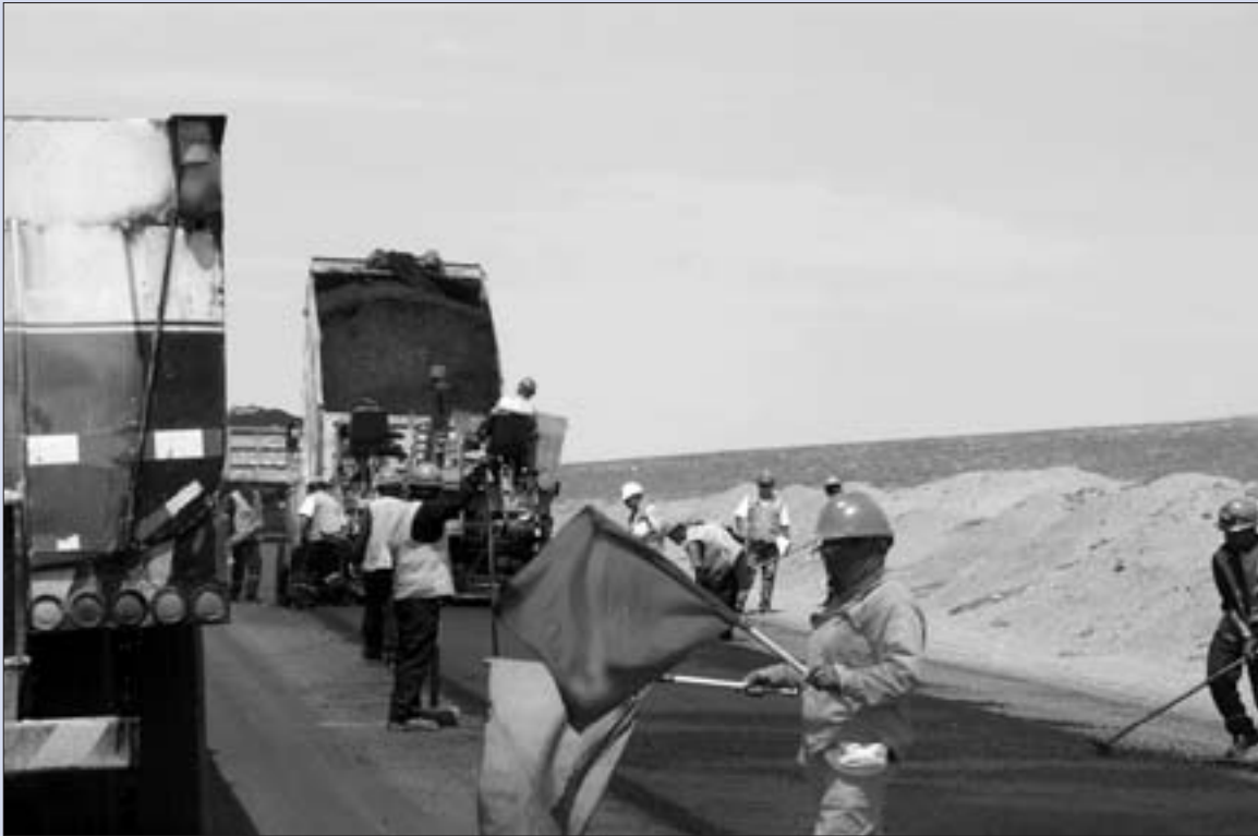
Crews working on a road in Peru. Photo courtesy of Jouni Martti Eerikainen.
