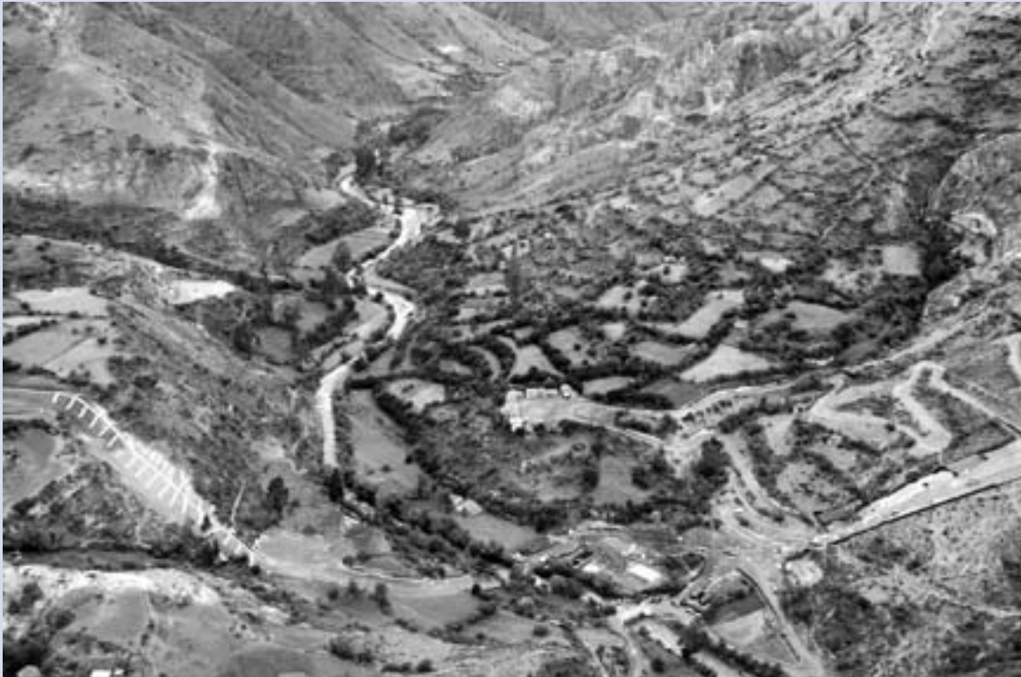
Construction of a pipeline in Peru. Photo courtesy of Jouni Martti Eerikainen.
