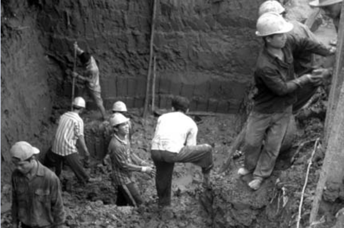
Construction workers excavating a canal-bed beneath a Hanoi bridge. Photo by Tran Thi Hoa, courtesy of the World Bank Photo Library.
