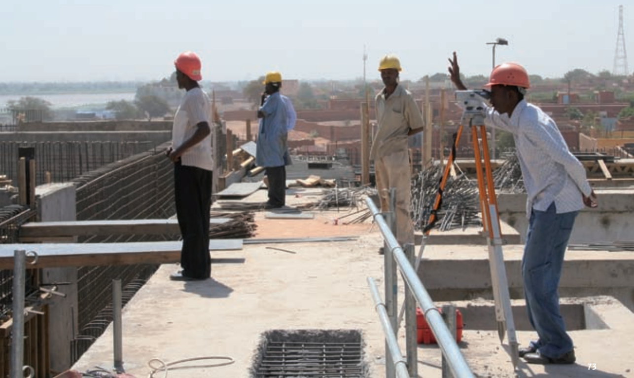
Construction of the Drinking Water Treatment Plant in Omdurman (Sudan)
