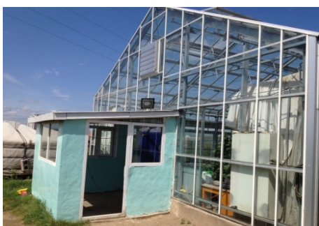
Picture 9. Two-layered door Installed by the PSARI
