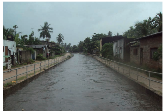
The drainage after the implementation of the Lunawa Environment Improvement and Community Development Project, Sri Lanka
