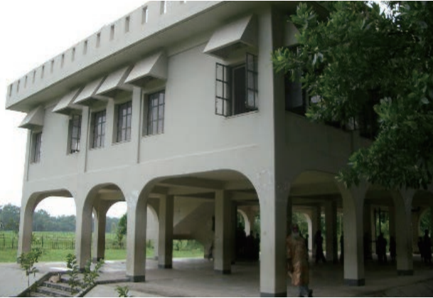
Cyclone Shelter in Chittagong (completed in 2005)
