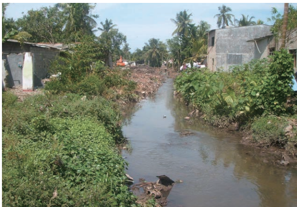
A drainage before the implementation of the Lunawa Environment Improvement and Community Development Project, Sri Lanka (photo taken in 2002)
