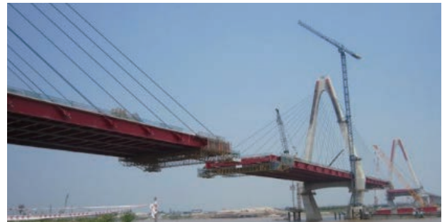
Nhat Tan Bridge under construction
