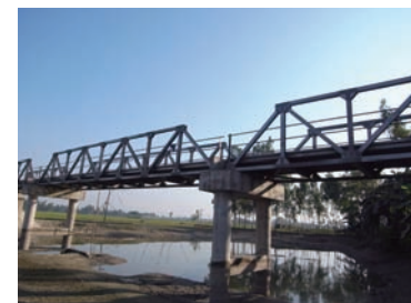
A bridge constructed in Sirajganj District
