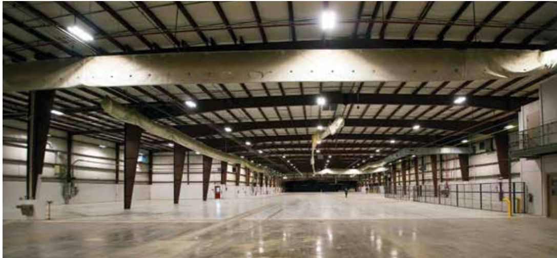
Refurbished Springhill, Louisiana, industrial park facility
