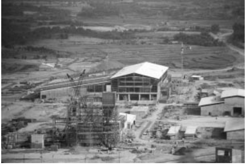
The project site in 1978. Photo: WP-System archive
