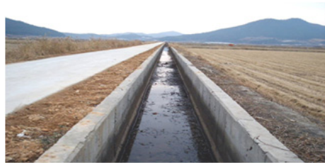
Irrigation Canal Farm Road
