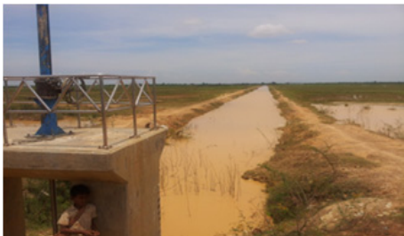
Irrigation & Drainage Canal
