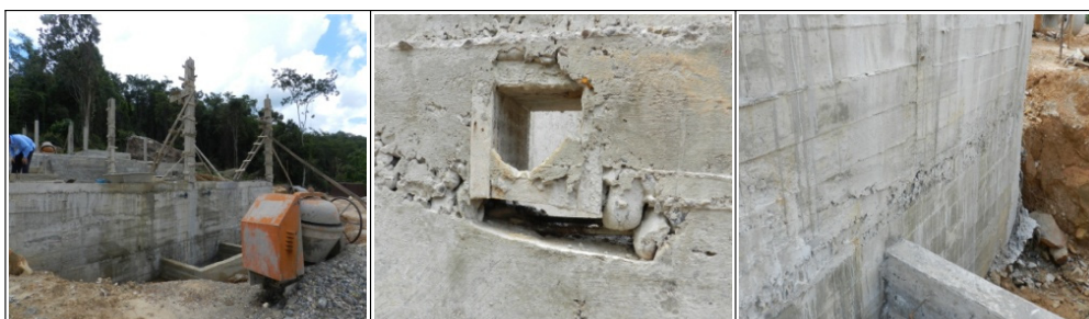
Photo 2-6 On-site visit to French-funded facility (construction by local company)
