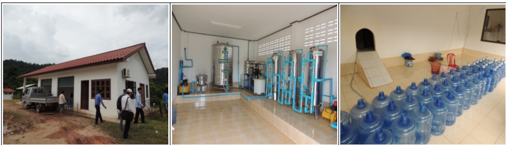
Photo 2-10 Drinking water facility in Bolikhan
