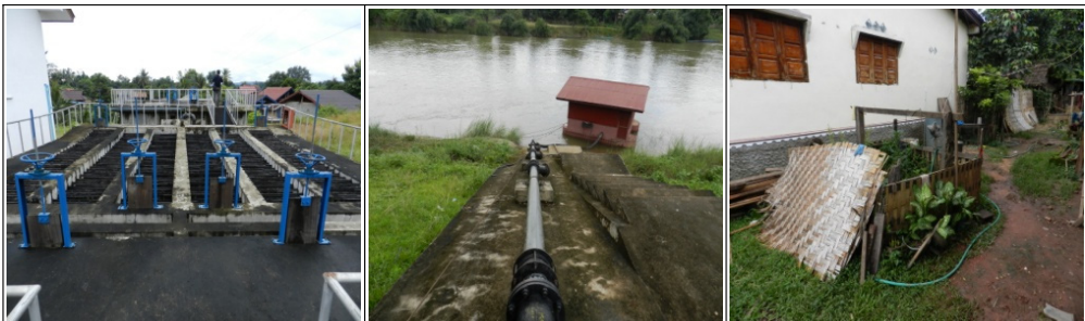
Photo 2-4 Project on-site inspection
