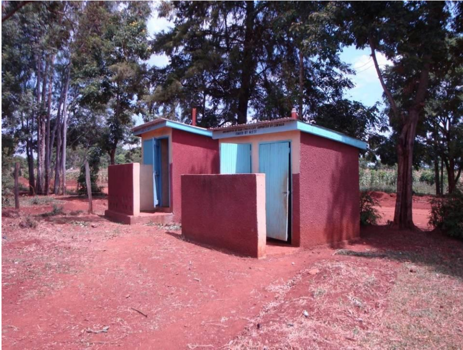
Figure 3 VIP latrines at Nasira School, Busia.
