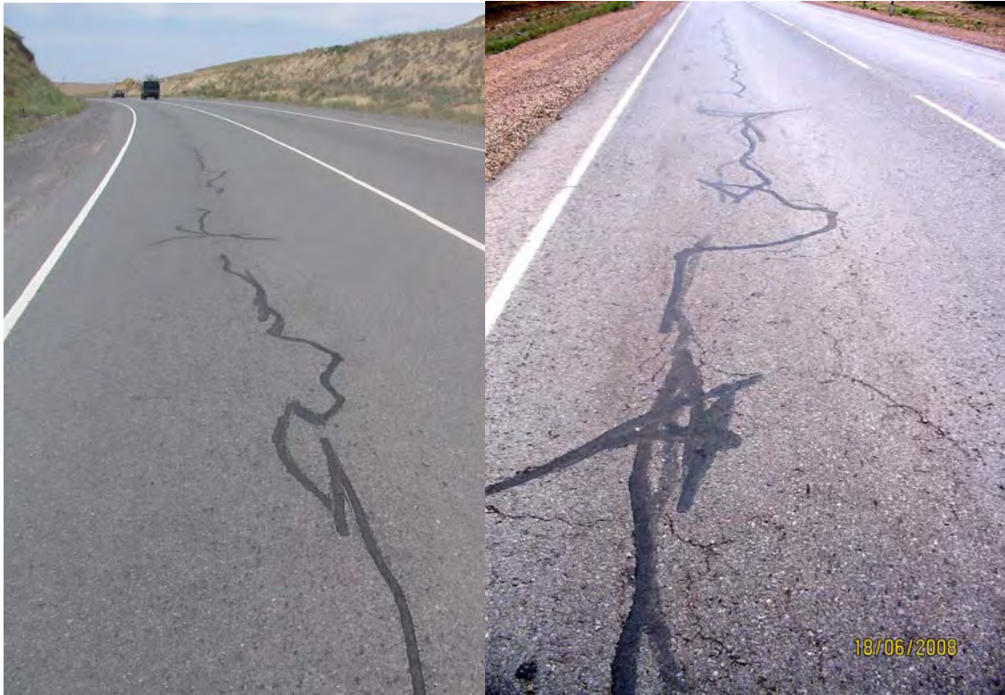
Photo A11.4: Poorly Sealed Shrinkage Crack
