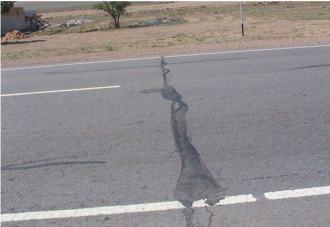
Photo A11.4: Poorly Sealed Shrinkage Crack
