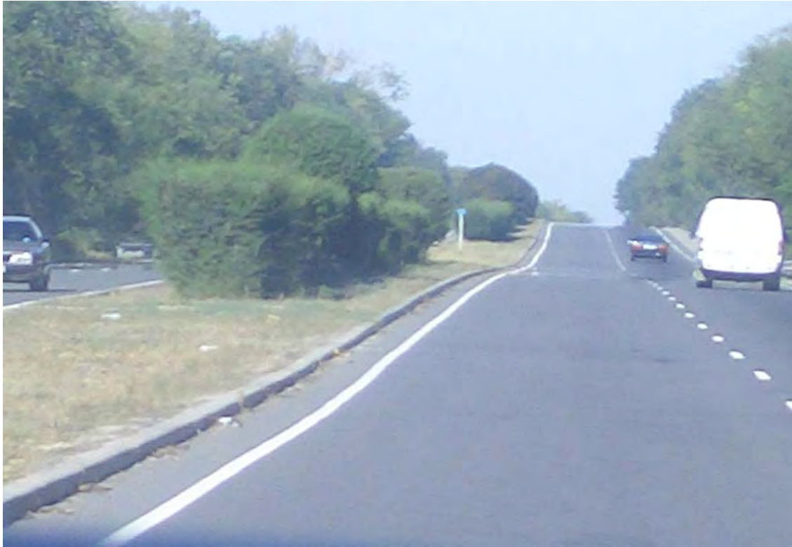
Photo A11.1: Contract 1, European Bank for Reconstruction and Development Section with Dual Carriage Way
